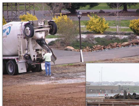
Figure 1. Chute washwater being dumped on the ground
